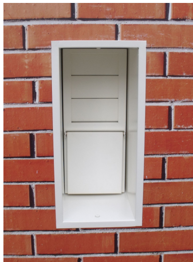
External View— the Top section is the Under Pressure Blades - Bottom section is the Over Pressure Cat Flap. The Weather Louvre is not shown for clarity.
